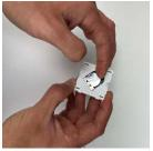
Step 5: Place the control back into the insert and then into the frame. Start at the bottom, inserting the wide prongs into the insert, followed by the two prongs closer together.
